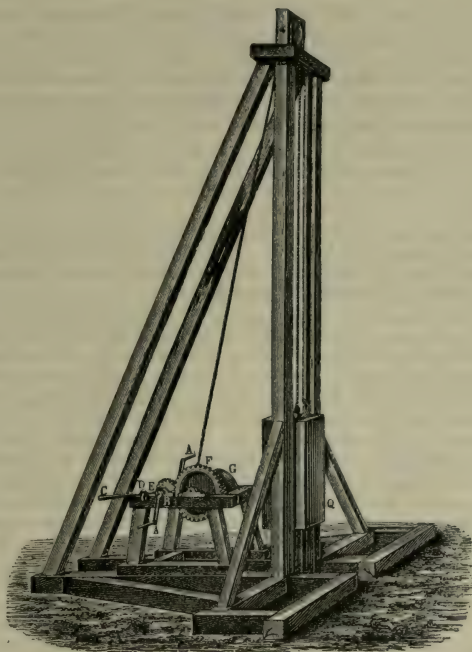
FIG. 146.—Pile driver (monkey engine).
